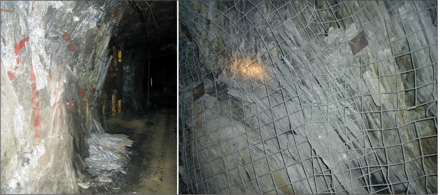
Figure 7.8 - Plate-like peices or flakes of rock - stress fracturing.
