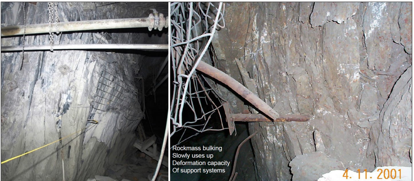
Figure 7.6 - Deformation of headings.
