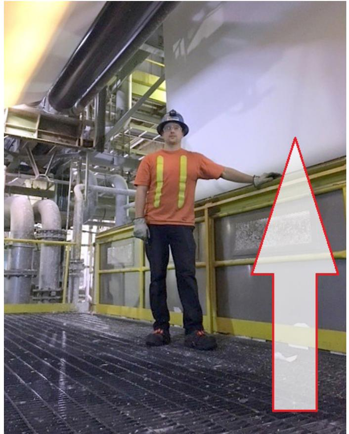
Guardrails are a passive form of protection to keep workers at a safe distance from hazards, such as:
