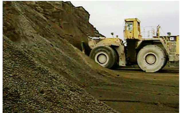
(a) Correct - equipment perpendicular to the face
