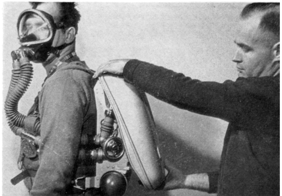
A mine rescue volunteer Gerry Tremblay dons a new Dräger BG174 breathing apparatus with the assistance of Mine Rescue Officer John Guthrie - 1968
