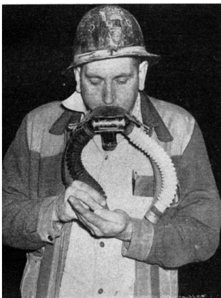
Testing the inhalation valve on the McCaa breathing apparatus - 1961
