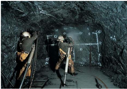
Manual Drilling, Bolting, Loading & Blasting
